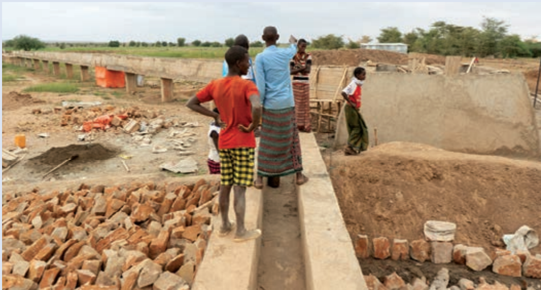
Image 60: A team of builders finalise the concrete irrigation canal in Hilaweyn II. © RSC/Raphael Bradenbrink, 2018
