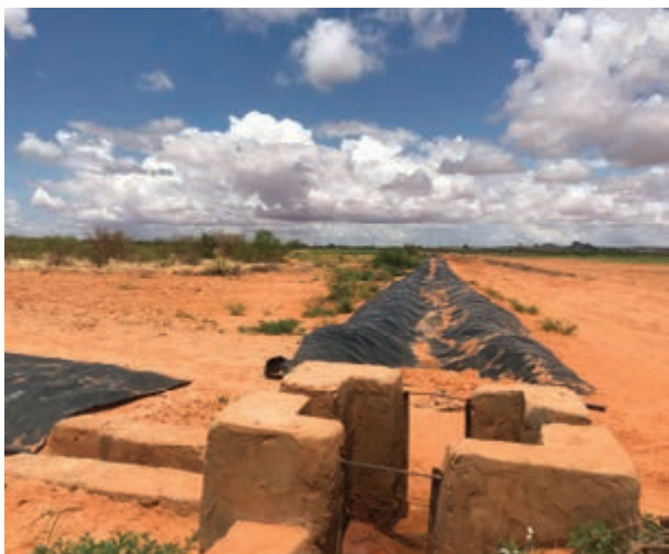
Image 24 (left): Geo-membrane canals are used to service farmland in Hilaweyn camp. © RSC/Andonis Marden 2019. Image 25 (right): Cooperative members stand on the reinforced concrete irrigation canal at a Melkadida farming site. © UNHCR/Eduardo Soteras Jalil, 2019
